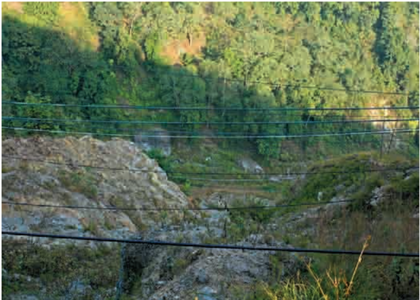
Pipes carrying water to the villages from Kuapani springs in South Sikkim
